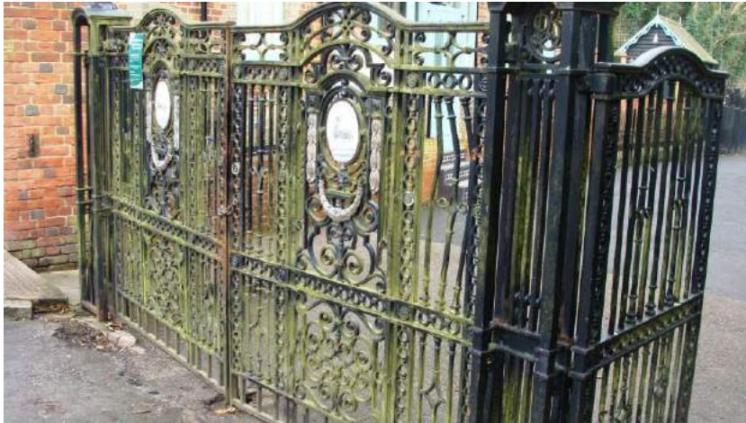
Picture 116. Decorative metal gates assumed to date from the earlier part of the 20th century are imposing and a strong feature in the street scene. Minor remedial works required.
