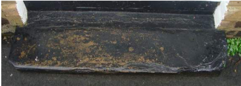
Picture 76. A well worn slate step to Port Vale terraced house.
